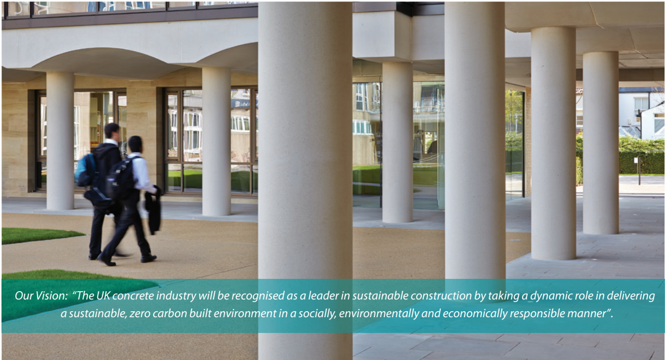
Precast concrete colonnades at St Paul's School, London. Image courtesy of Nicholas Hare Architects © Alan Williams Photography
