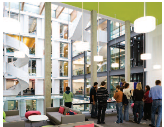
The Informatics Forum at Edinburgh University, designed by Bennetts Associates, has exposed concrete offering high thermal mass and has achieved a BREEAM rating of 'Excellent'.
