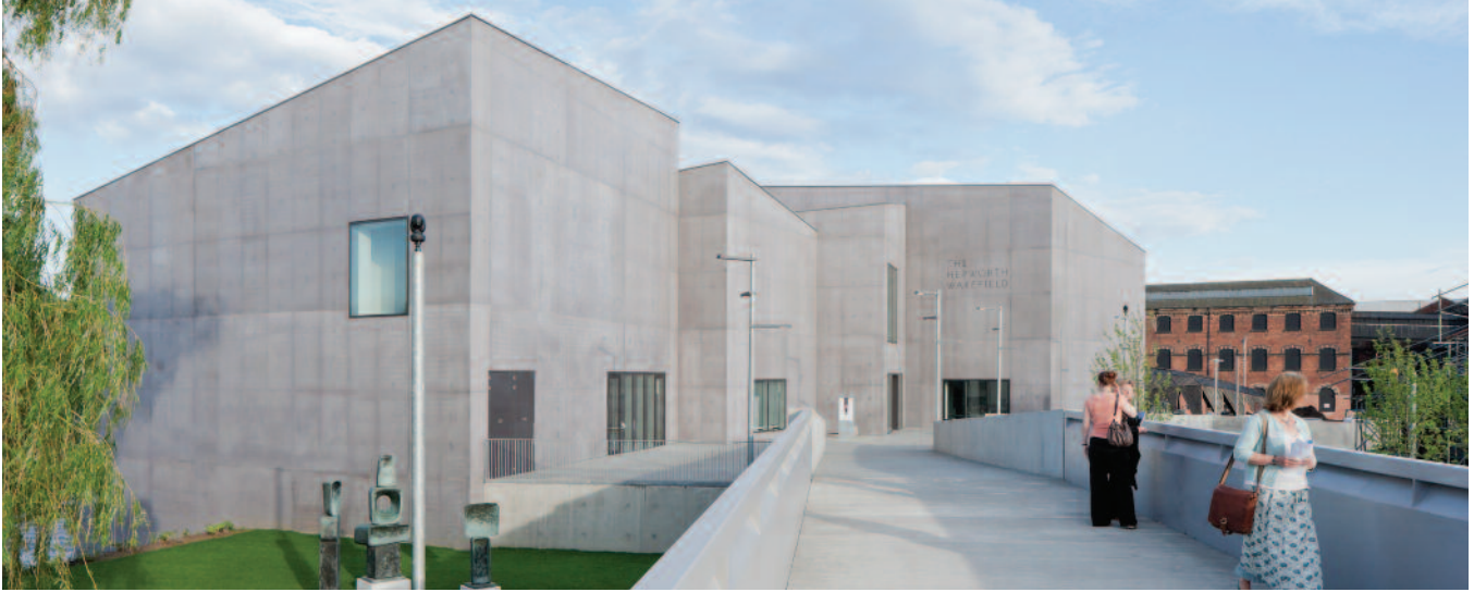
Completed in 2010, the award-winning Hepworth Gallery is constructed using self-compacting pigmented concrete.
