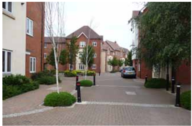
Permeable concrete and concrete block paving (shown above) can be used to reduce, attenuate and treat surface water as part of a sustainable drainage solution (SuDS). The water can then be used within the landscape to enhance biodiversity.
